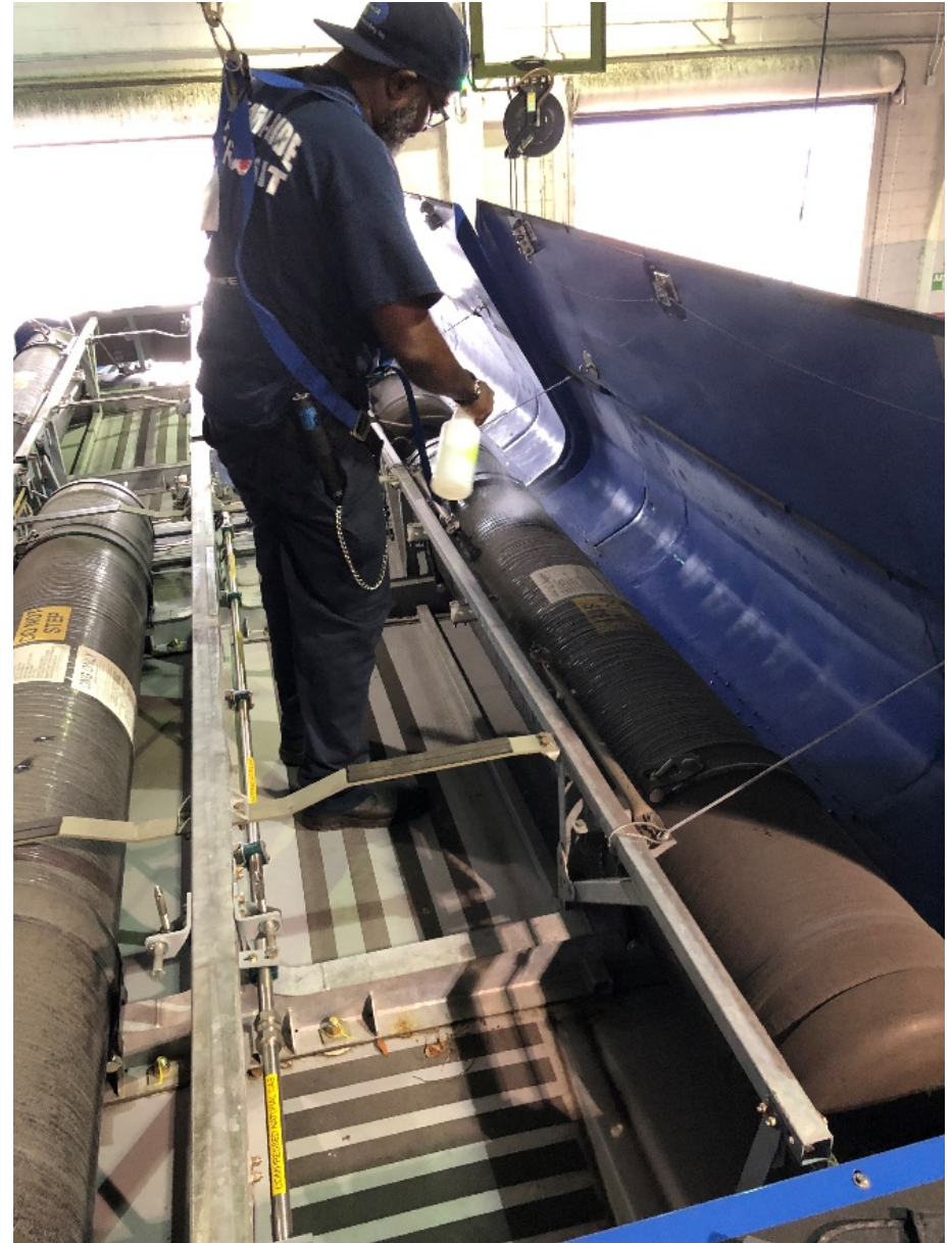
6. Inspector spraying surface of CNG storage tank with soapy water to clean surface of tank. A clean tank surface is required to perform a visual inspection of the tank.
