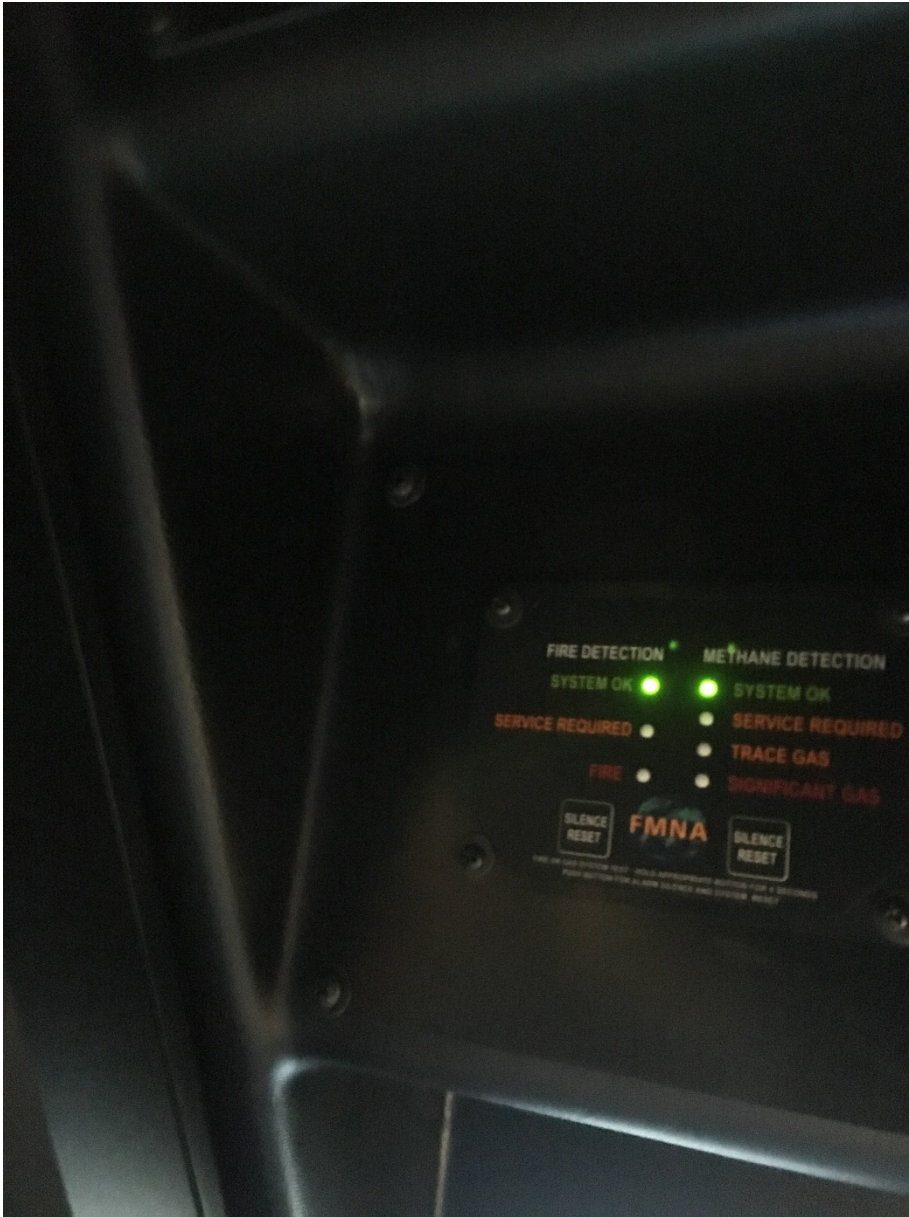
9. FOGMAKER Fire Detection and Methane Detection alarm panel in New Flyer bus located in left over-head panel. Both system lights are “green” indicating “SYSTEM OK”
